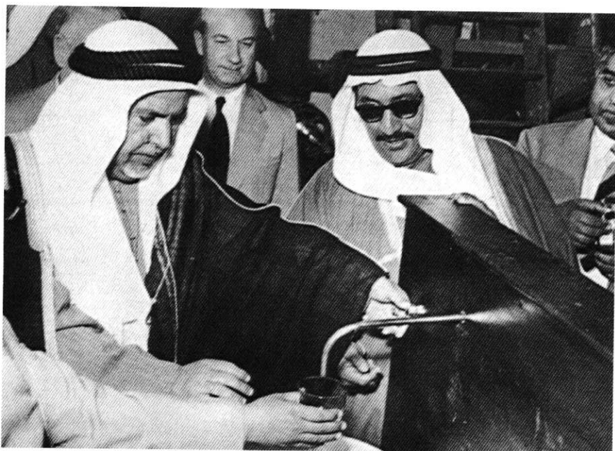
Plate 14. Sheikh Abdullah Al Salem and Sheikh Abdullah Mubarak drinking a cup of water at Kuwait's first desalination plant, Shuwaikh, March 1953.
